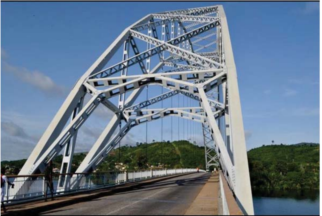
Adomi Bridge – The gate to Volta Region
